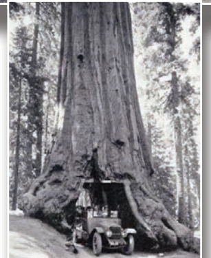
Going through the Wawona Tunnel Tree, Mariposa Grove, CA
